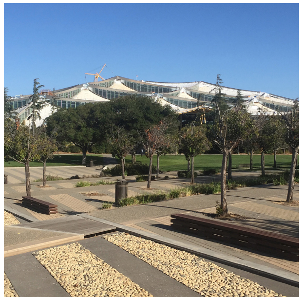
New Google Headquarter, Charleston East, under construction
