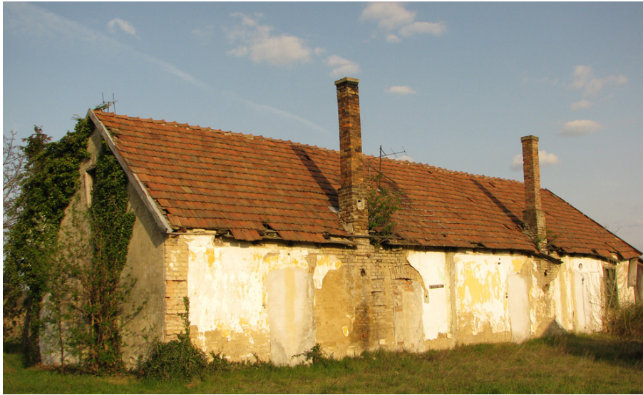
Fig. 5. Old vernacular structure (a relic before the development plans of 1960)
