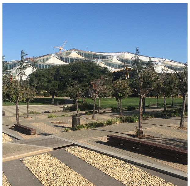
New Google Headquarter, Charleston East, under construction
